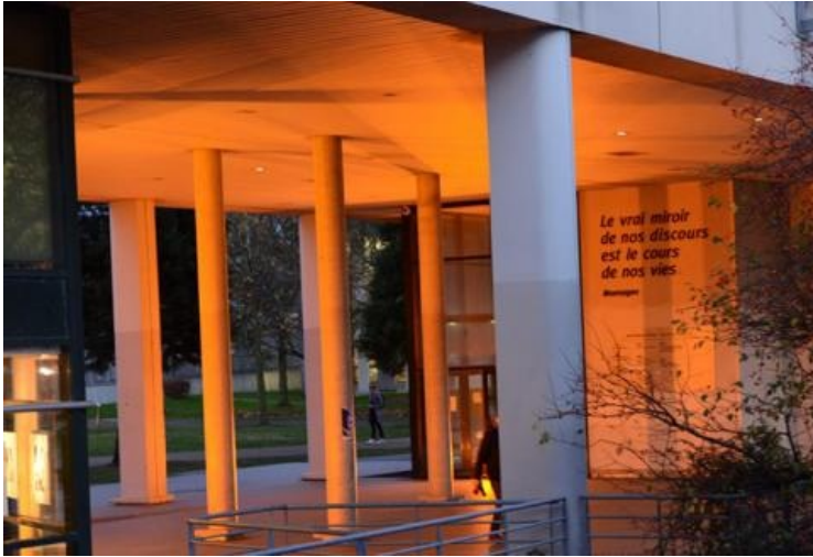
The Presidency Building of the Villejean campus lit up for Orange Day
